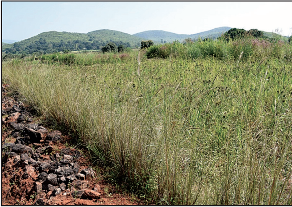
Bio engineering (stonebunding+grass) measures
