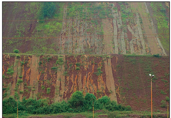
Geo jute cover with grass planting in mine spoiled area
