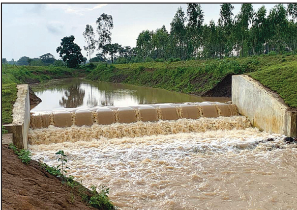
Masonry check dam
