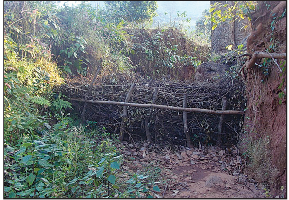
Brush Wood Check Dam (BWCD)
