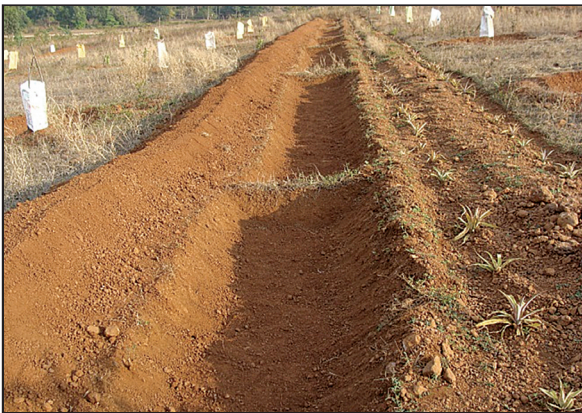
Trench cum bunding with Pineapple barrier
