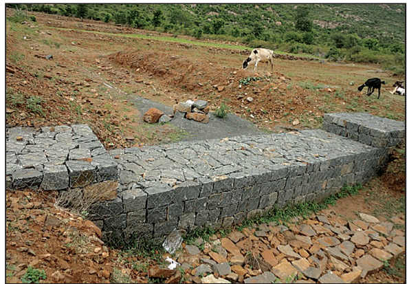
Gabion check dam
