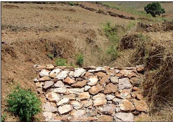
Loose boulder check dam
