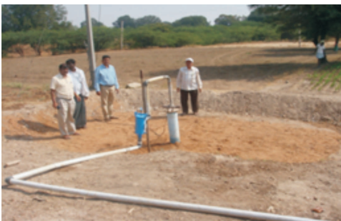
Stage 4 : Sand filling over nylon mesh
