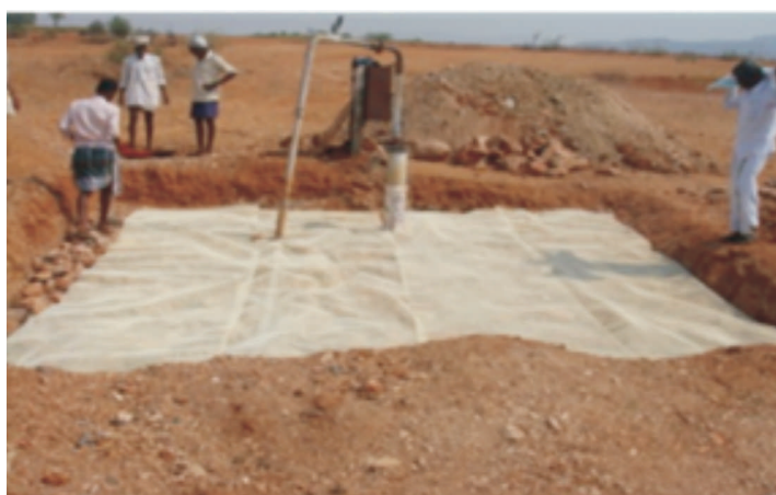
Stage 3 : Spreading nylon mesh over stone layer
