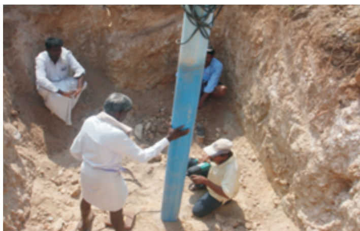
Stage 1 : Excavation of pit
