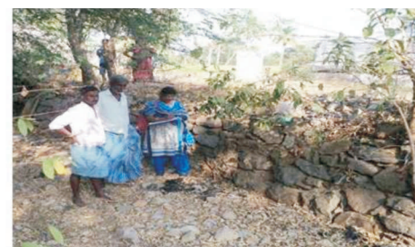
Stone paving in gully banks for erosion control
