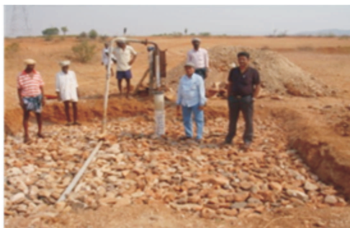
Stage 2: Stone filling in pit
