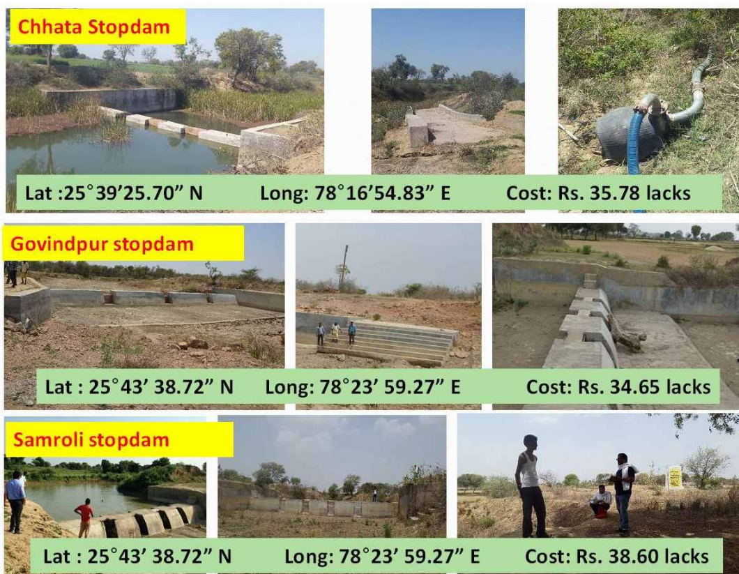
Fig.- 4: Identified Stop dams constructed under Bundelkhand package, Datia
