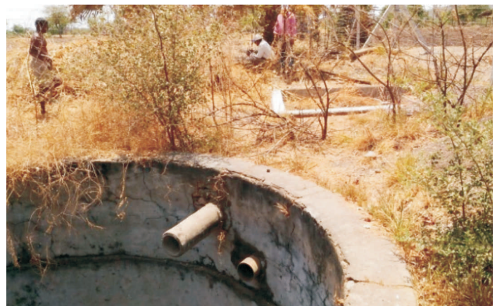
Fig.-22: Recharge filters constructed in the farmer's field
