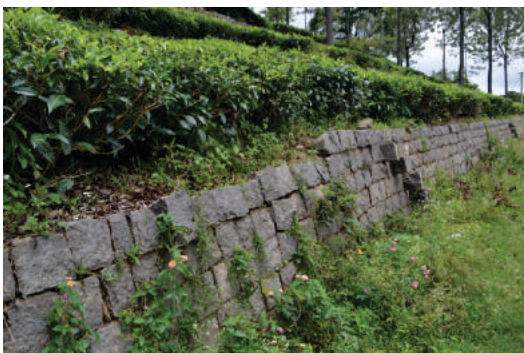
Terrace support wall in tea garden
