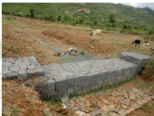
Gabion check dam
