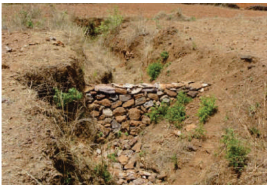
Loose boulder check dam for gully control
