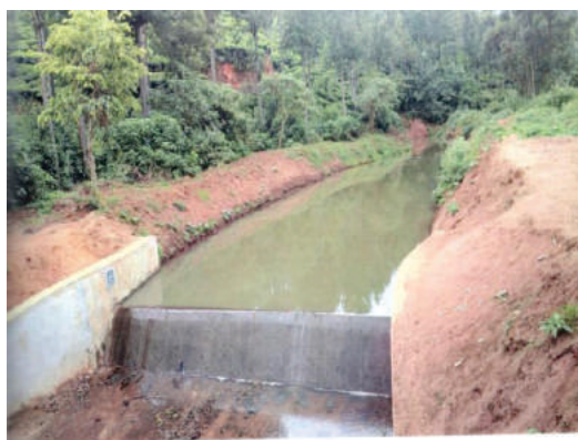
Masonry check dam
