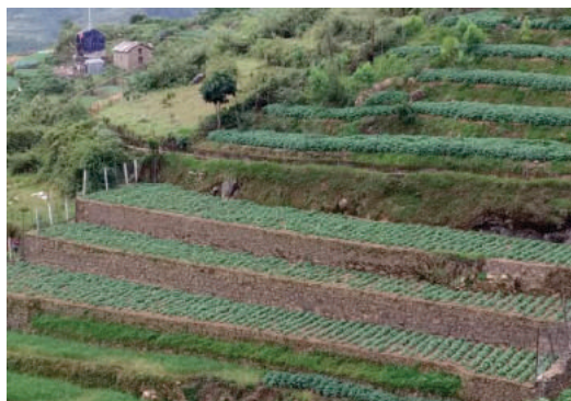
Terrace with stone support wall
