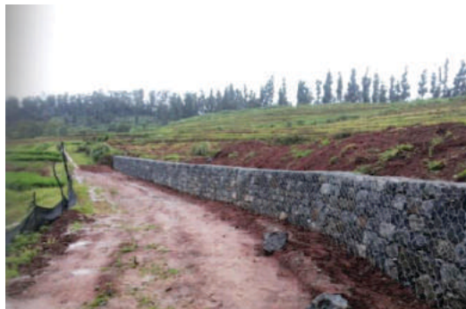
Gabion terrace support wall
