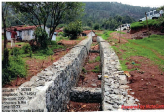
Gabion stream bank protection wall
