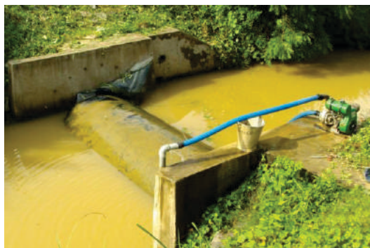
Rubber check dam
