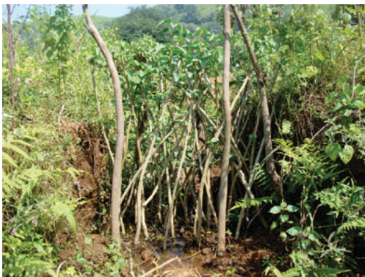
Live check dam
