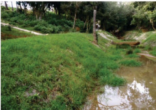
Gully erosion control by geo jute with grass cover
