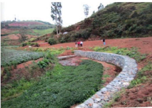
Gabion terrace support wall
