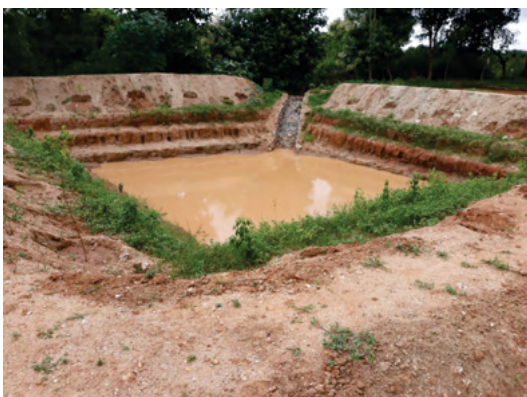
Farm pond constructed in red soils to harvest rainwater for life saving irrigations in Chamarajnar district
