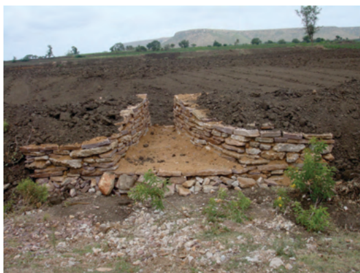
Waste weir in black soil for drainage of excess runoff in Koppal district
