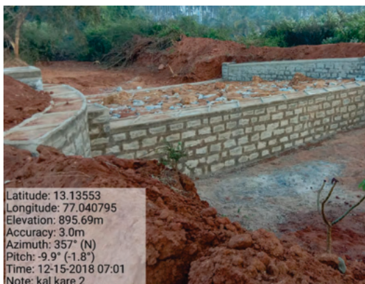
Masonry check dam to store runoff, erosion control and providing supplemental irrigations to arecanut plantations in Tumkur district.
