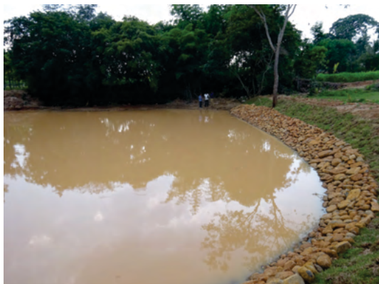
Gokatte for capturing rain water for facilitating drinking water to livestock and ground water recharge in Tumkur district.
