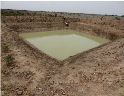
Farm pond constructed in black soils to harvest rainwater for life saving irrigations in Koppal district
