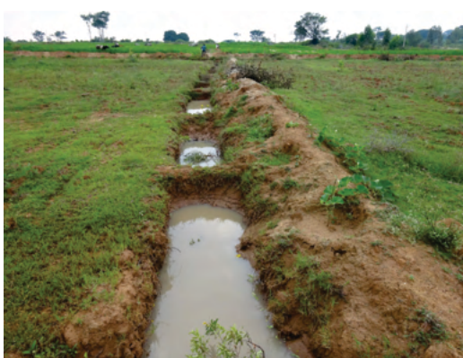
Trench-cum-bund for in-situ moisture conservation and erosion control in Tumkur district
