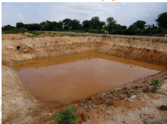
Farm pond in red soils constructed to harvest rainwater for life saving irrigations in Koppal district
