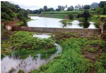
Series of percolation dams constructed (February 2009 to March 2016)
