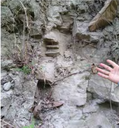
Sedimentary rocks (siltstone and shale) which range in age from Miocene to loosely consolidated sediments of recent age in Bishalgarh block
