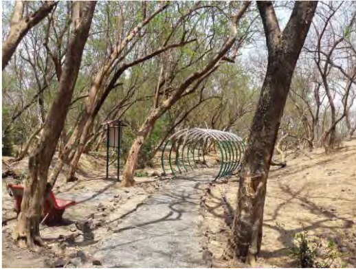
Walkways under Construction
