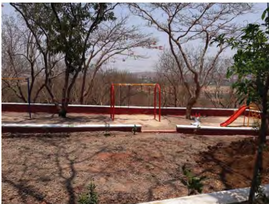
Children Playing Area under Construction
