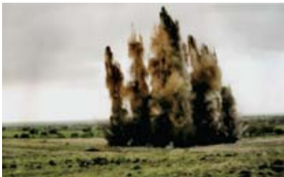
Blasting in the bore wells
